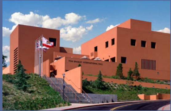
The Bradley International Hall
